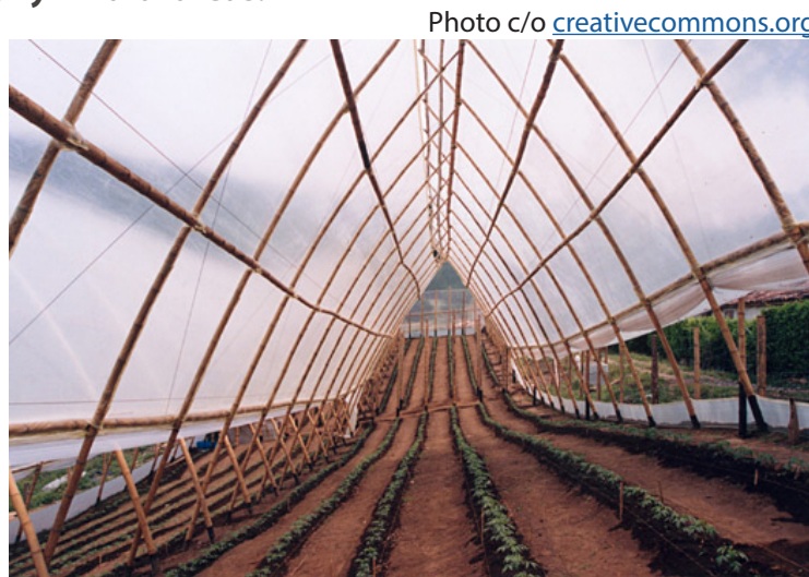
Figure 5-4. Construction with poles (instead of finished lumber) is common in tropical countries, especially in rural areas.
