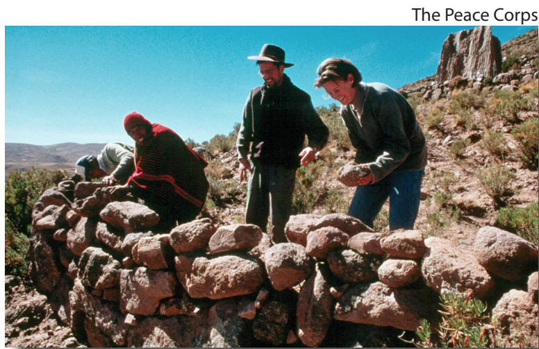
Figure 4-9. A Loose Rock Wall Barrier
