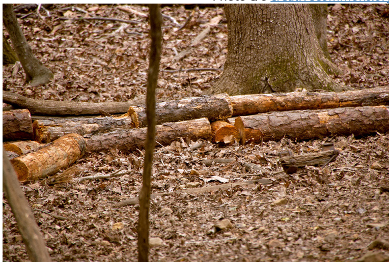
Figure 4-8. Erosion Control - Dead Barriers Made of Tree Logs
